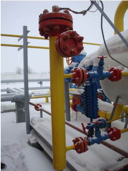
Two-points level sensor TLA on the condensate tank Level sensor UTS on the outside station of the Preparation System of the Fuel Gas
