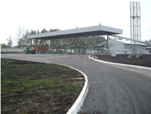
Loading facility of petroleum products
