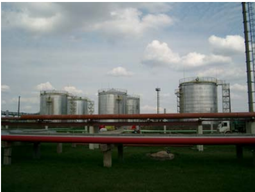
Overview of the reservoir park of scouring installations sensor on the reservoir with water containing oil
