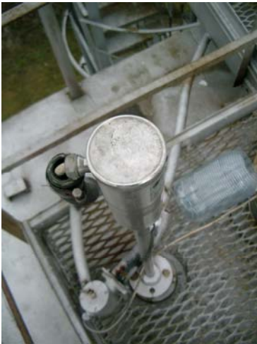
Level Sensor on the reservoir
